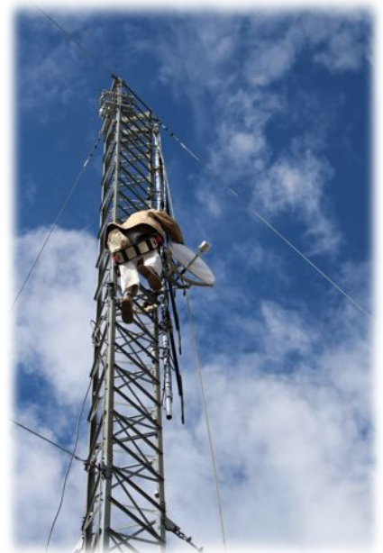
Installing microwave dish
